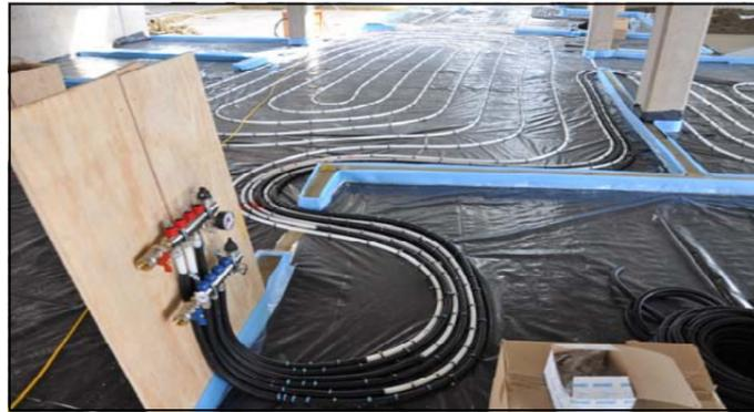
Underfloor heating is currently being installed in some parts of the building.
