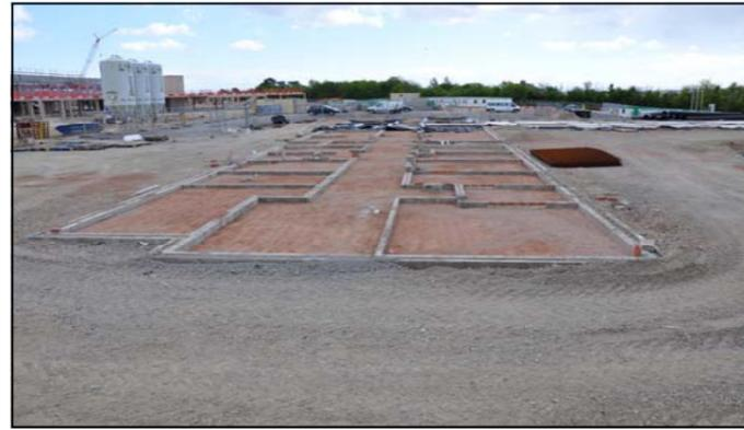
Foundations and initial setting out for the Respite Centre were complete during May, allowing block work to begin.
