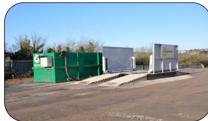
A wheel wash is now in place which is large enough for all vehicles on site, including wagons and delivery lorries. All vehicles leaving site will go through this before driving onto the public highway.
