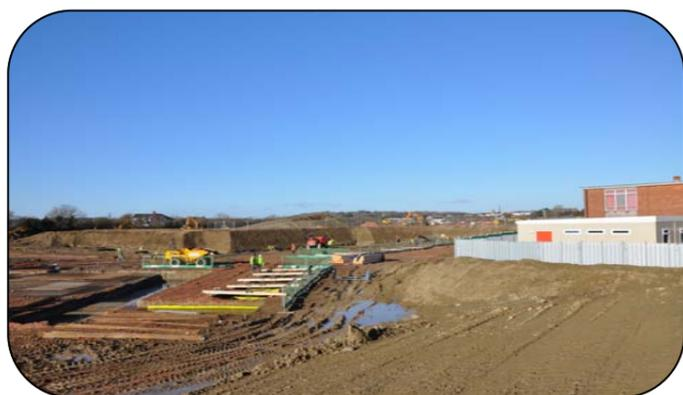
The retaining wall has been prepared to support the separate levels required. This will be supported by a reinforced concrete frame which we have begun pouring.
