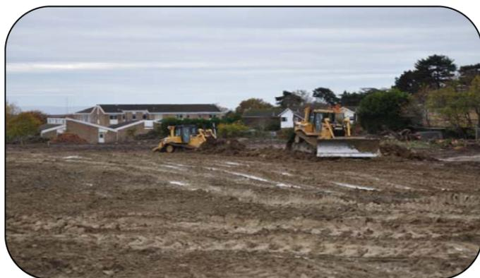
A lot of machinery has been required to dig the levels needed across the site. This machinery uses satellite tracking technology to ensure correct levels are achieved.
