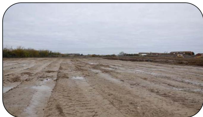
A similar view of the site following the turf and topsoil removal. No material has been removed from the site and topsoil will be reused later in the project.
